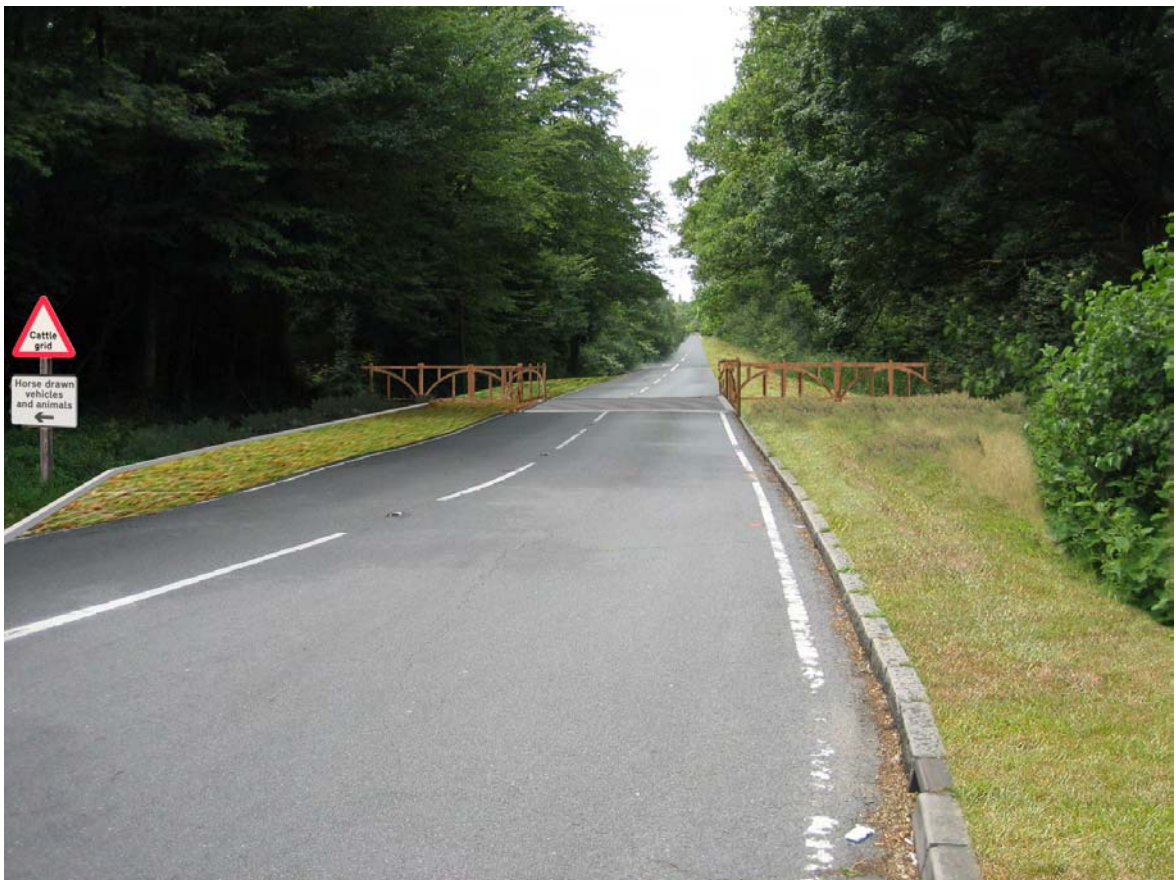
A photomontage of a proposed cattle grid location at the eastern end of Rangers Road, Essex near the junction with the A104 (looking west along Rangers Road). The photomontage shows the bypass gate and access track along the left-hand-side.
